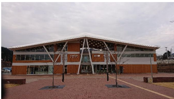
New Onagawa Station
